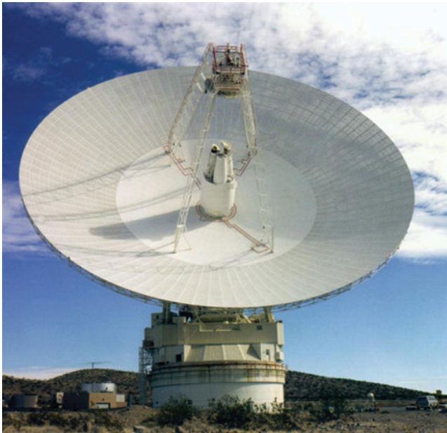
FIGURE 11.37 Seventy-meter Goldstone steerable parabolic dish antenna used in NASA's Deep Space Network. (Photo courtesy of NASA.)
